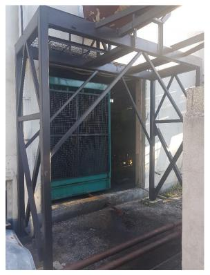
Figure 4 Cummins QSK60 set outside view
