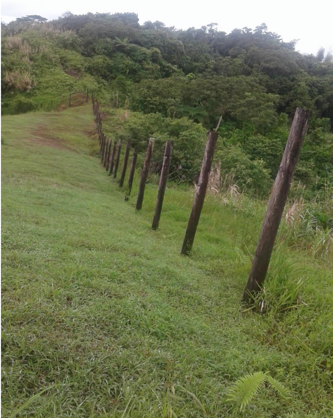
Fig1. Section of fence where chain link is missing
