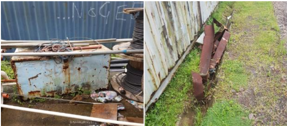
Figure 14 : Scrap outside the Power station
