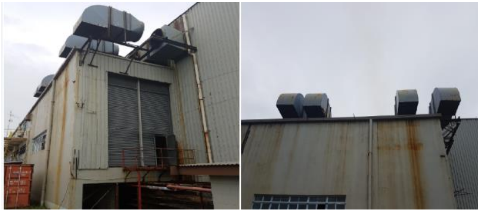
Figure 6 : Old 33kV switch gear room scrap 1
