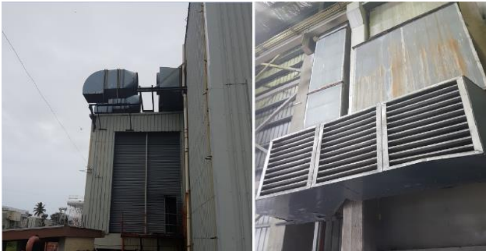
Figure 7 : Old 33kV switch gear room scrap 2
