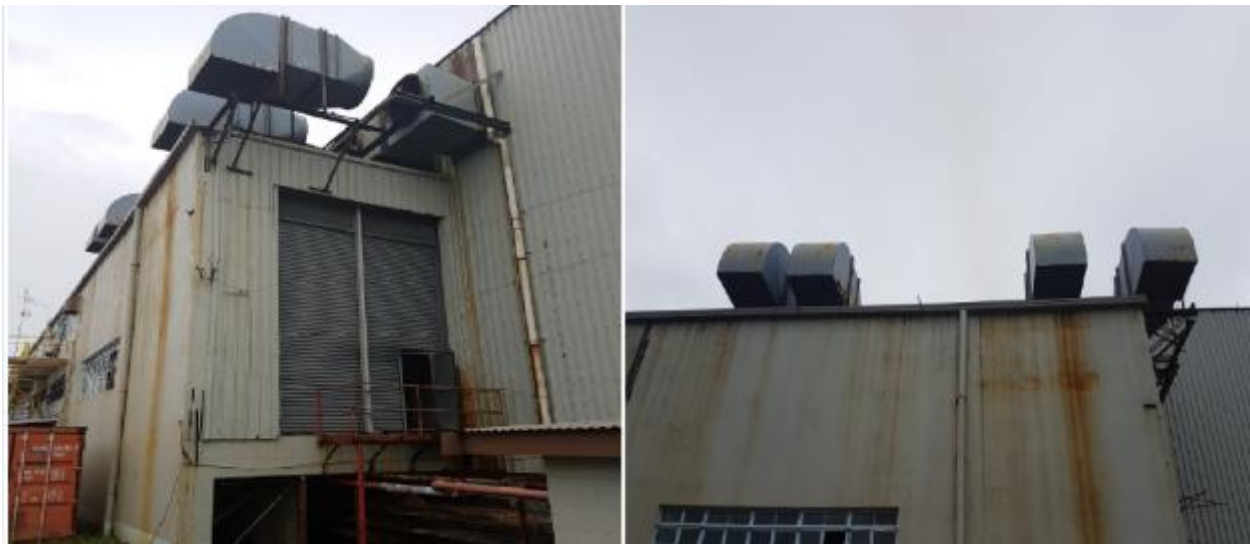
Figure 6 : Old 33kV switch gear room scrap 1
