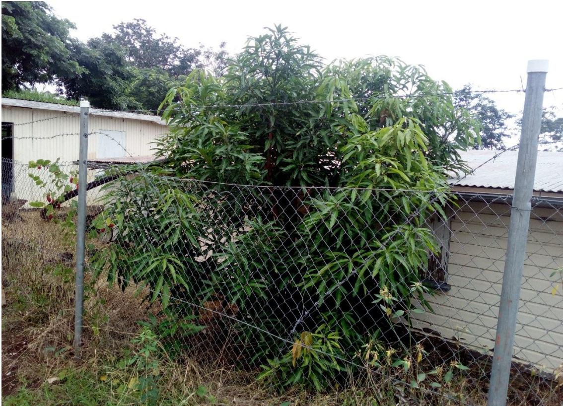
Fig 4. Broken barbed wire
