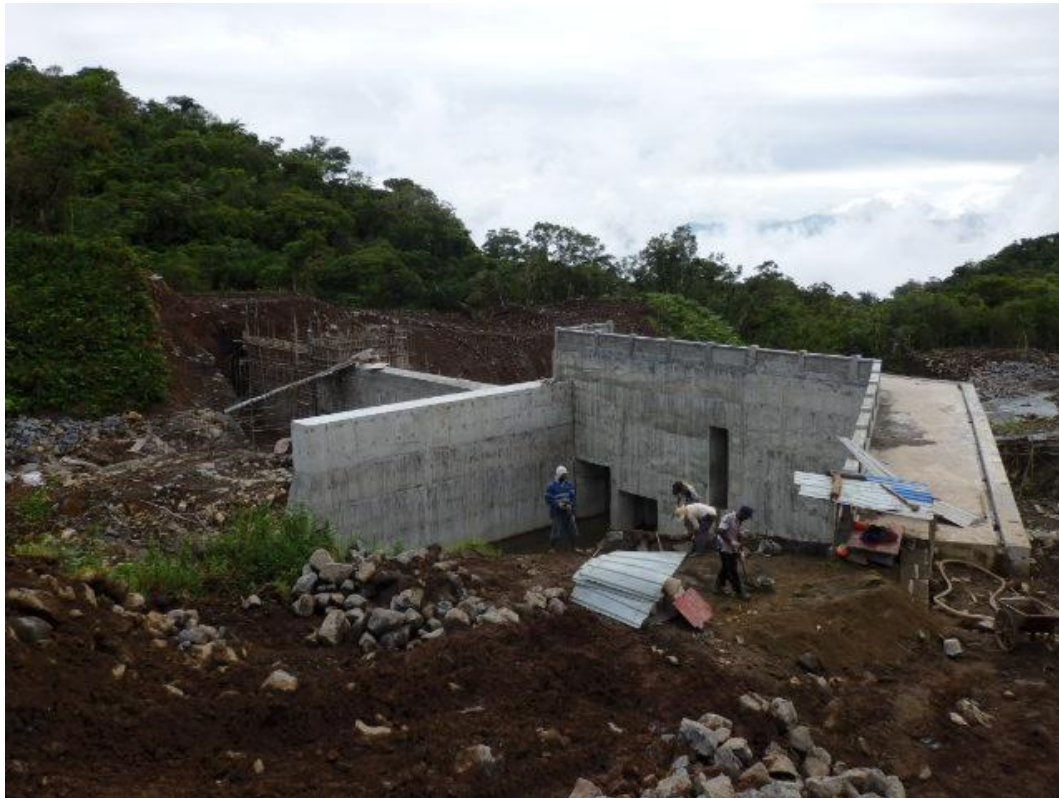
Somosomo Hydropower Scheme Weir Under Construction.
