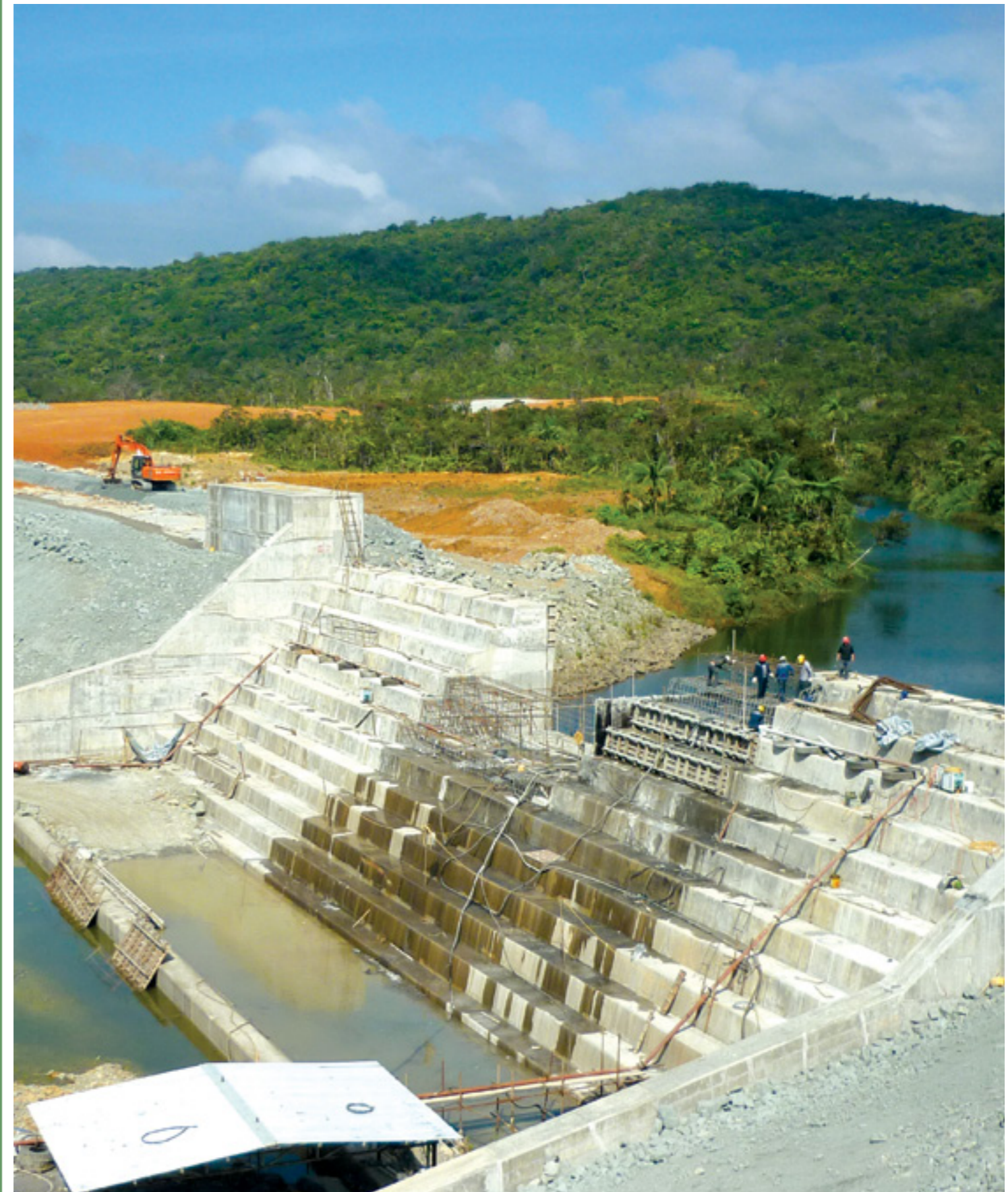
The Construction of the Wainisavulevu Weir Raising Project progressed according to work schedule for 2014. The project is expected to be completed in 2015. When completed it will produce additional 10 million units of electricity per year equivalent to a diesel savings of around $4M per annum. FEA invested around $40M to increase the height of the existing Wainisavulevu Weir.
