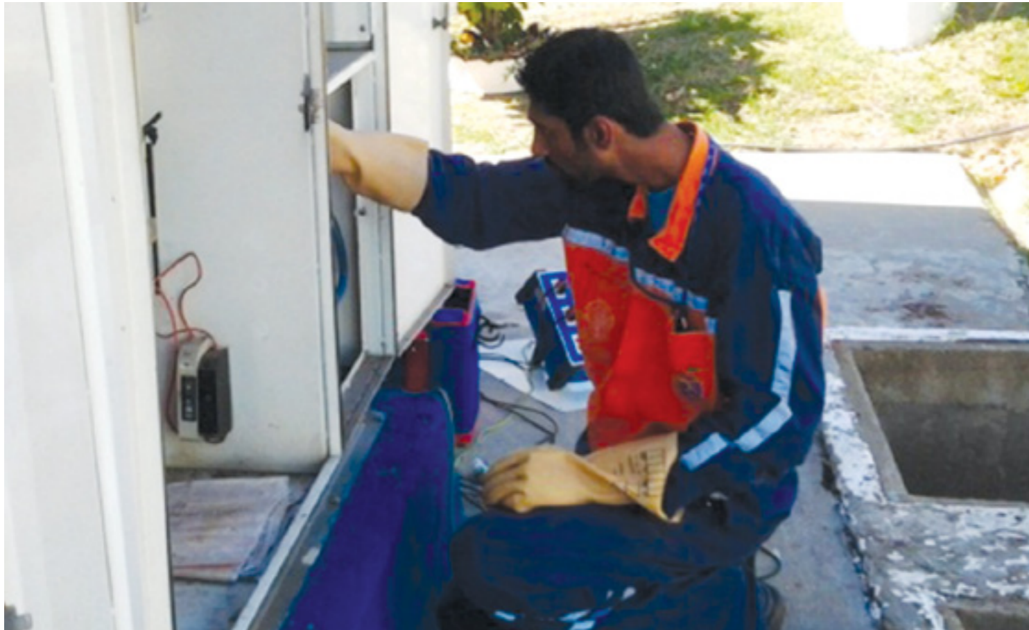
FEA Metering Technician carrying out metering system re-calibration at Water Authority of Fiji in Lautoka. This is to ensure that the customer's meters were functioning properly and recording correct consumption.
