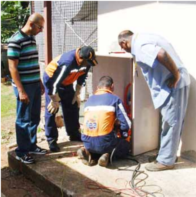
FEA Metering Team carrying out metering system re-calibration at Future Farms in Ba.
