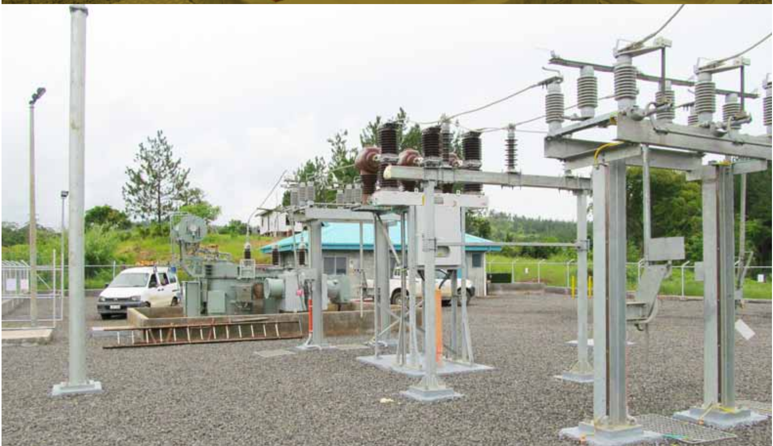
The newly established 11kV/33kV Zone Sub-station at Cawaira Power Station in Labasa which was constructed as part of the Dreketi Electrification Project.
